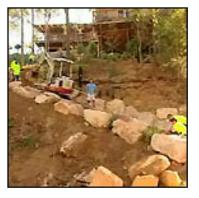
We contacted an excavator/operator who was experienced in placing boulders. We then cleaned out loose material on site and established a firm base for the first row of boulders. We had already ordered 100 tonnes of boulders to retain the high and loose sections of the site. This was achieved by methodically placing boulders in position and juggling sizes to fit. The boulder wall has a batter - the wall is stronger when slightly angled towards the material to be retained.
